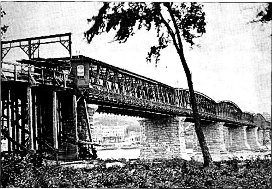
FIGURE 4. Looking towards Kansas City at the wood/iron trusses and the trestle.
